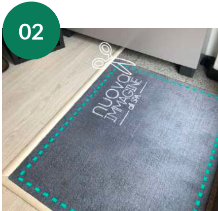
PREPARAZIONE AREA E TAGLIO ZERBINO PREPARATION OF THE AREA AND CUTTING
