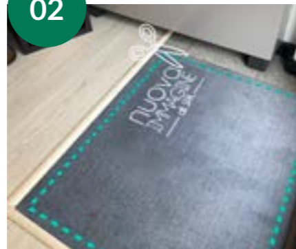
PREPARAZIONE AREA E TAGLIO ZERBINO PREPARATION OF THE AREA AND CUTTING
